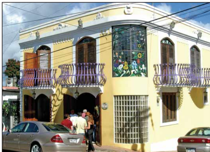
Dr. Sanchez helped design the Fondita Divino Niño Jesús rehab center in Aibonito, Puerto Rico, for drug and alcohol abusers.
